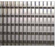
Plated metal that is welded into a grid can chip and peel over time due to expansion and contraction.
