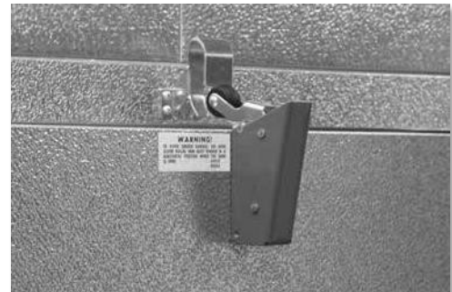
Roller Too High
