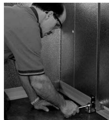
Attach slam brace with fastener provided
