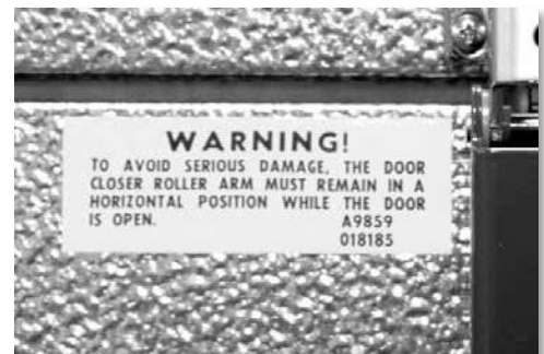
A warning label is affixed to the door section as a reminder.
