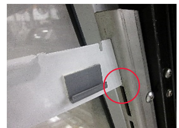
Bottom notch installed (no gap)
