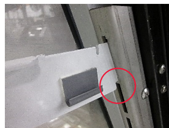
Top notch installed (gap)
