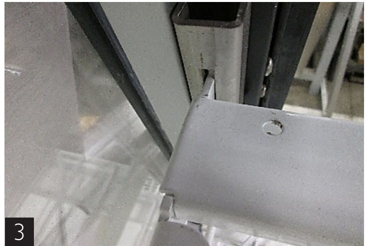
3 Light assembly installed on shelf support
