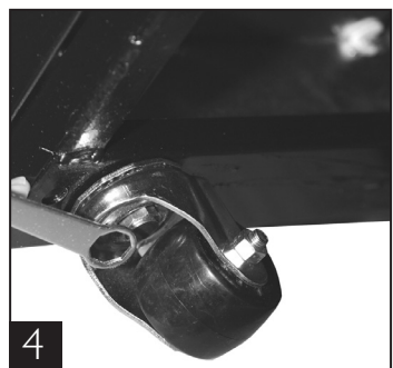
4 Tighten castor in position with castor wrench.
