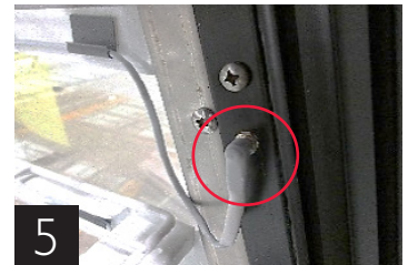
5 Light cord installed
